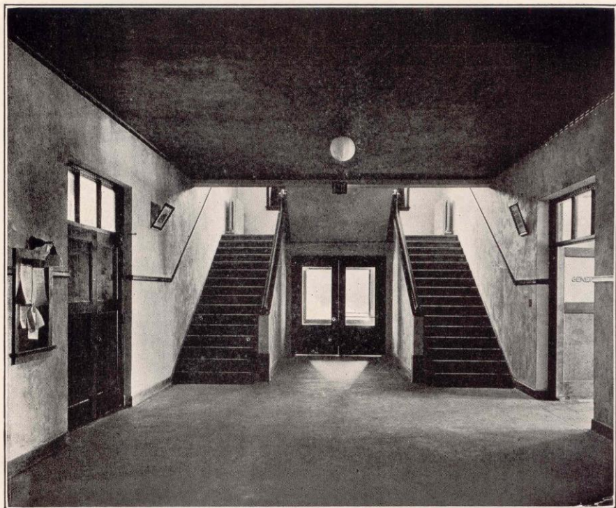
Interior View of Front Entrance and Stairway
